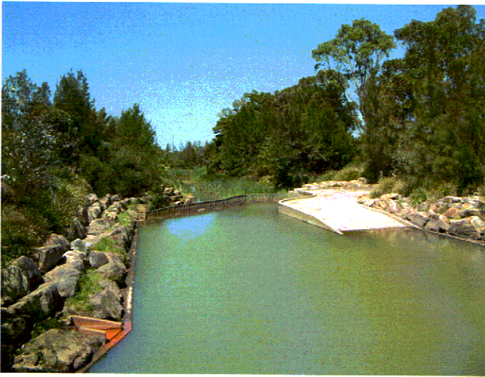
The Gross Pollutant Trap near Harbord Road
