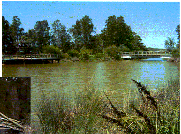
Above: The new bridge and viewing platform
