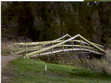
Below: The old Park Street bridge removed in 2000
