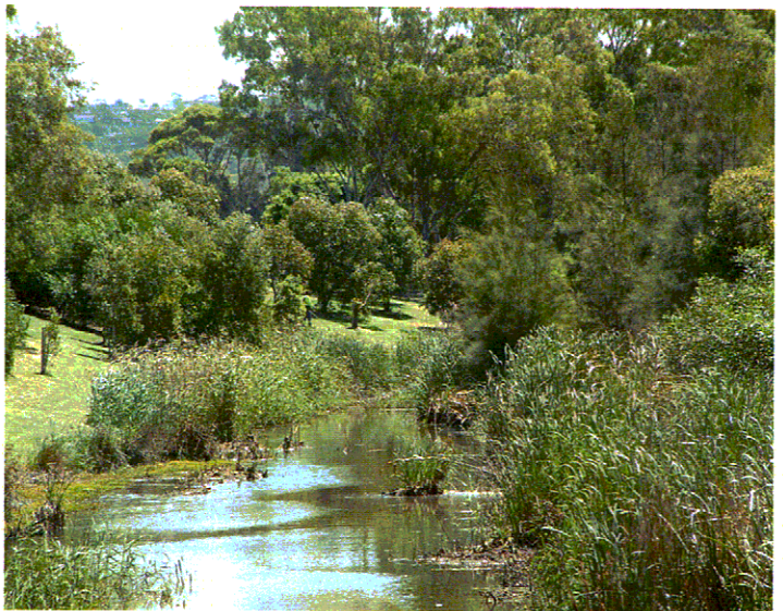
Part of the Stage 3 works to Greendale Creek
